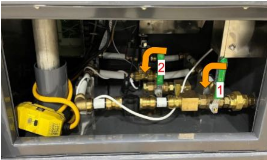
Figure 13) Turning Off Both Water Inlet Valves
