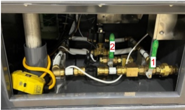
Figure 12) Open the Inlet Water Valve
