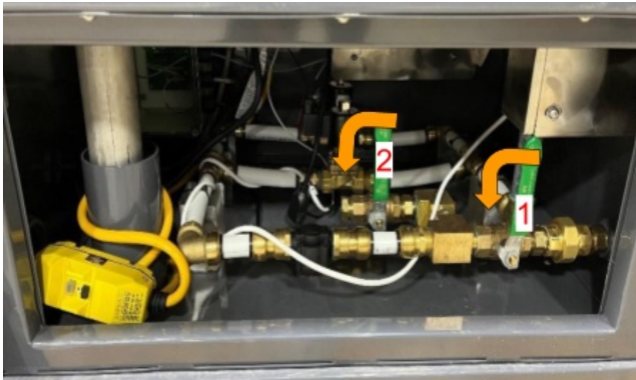
Figure 13) Turning Off Both Water Inlet Valves
